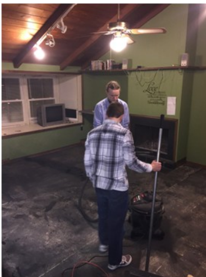
Getting ready for the new carpet!
